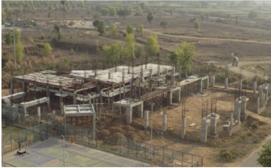
Gymkhana: 35% complete (RCC work is in progress)
